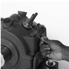
Figure 6 - RTL Circulating Oil Inlets
